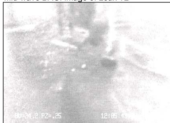
Mid-wave BAGI image of Leak T2
