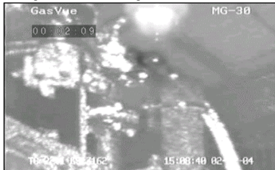
Long-wave BAGI image of Leak M7
